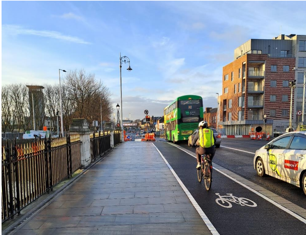
Image 3. C2CC - Works progressing well on Annesley Bridge inbound
